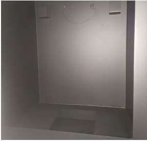
1. Clean fire chamber.
